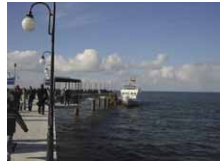
The view of new pier in Międzyzdroje
